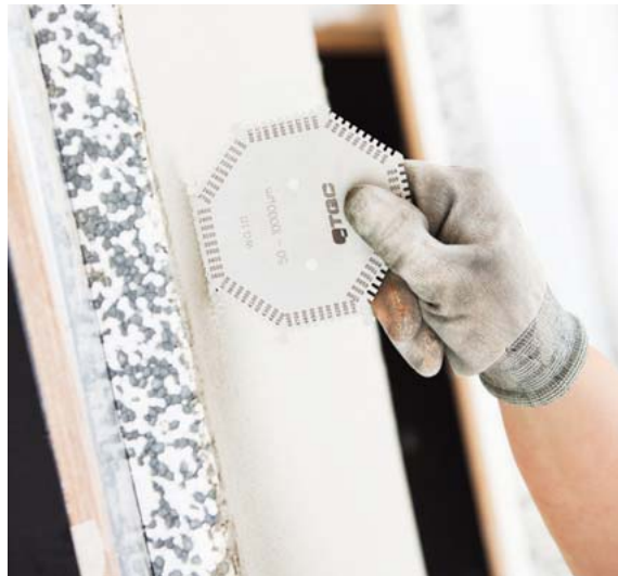
Layer-thickness measurement on reinforcing in the DAW Facade Technical Centre.
