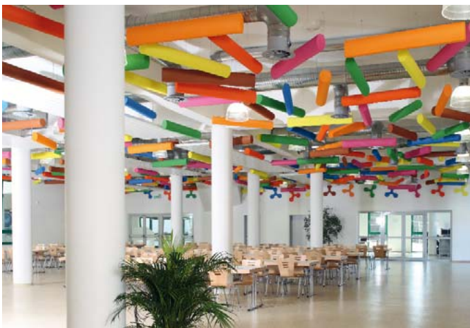
Noise nuisance sustainably reduced – a pleasant acoustic room climate was produced by the use of Melapor elements in the refectory of the school centre in Wesseling.
